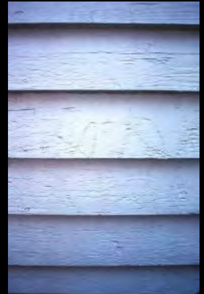
Chemical strippers can raise the grain of the wood
