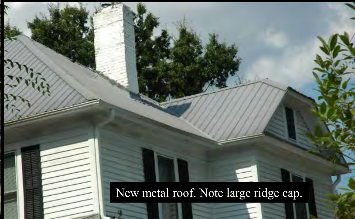
New metal roof. Note large ridge cap.
