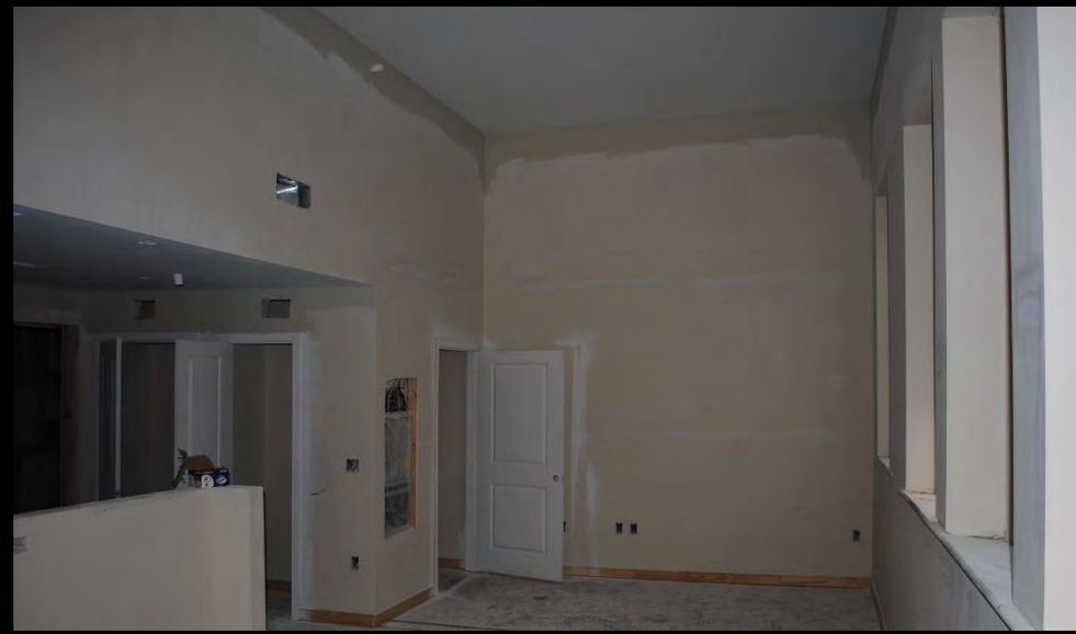
Unit 1D - Later drop ceilings were removed. The volume of space was retained along the exterior wall, but apartments received a one-hour fire rating by installing sheetrock over the plaster walls and wood ceilings and Gypcrete was floated atop the wood floor.
