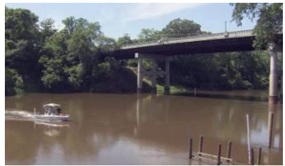
Comprehensive Land Use Plan; Cape Fear River, Bragg Blvd, Ramsey St., Murchison Rd. & Raeford Rd. Plans
