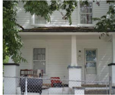
513 School St. Before/after photo
