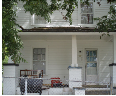
513 School St. before/after photo
