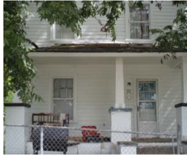
513 School St. before/after photo
