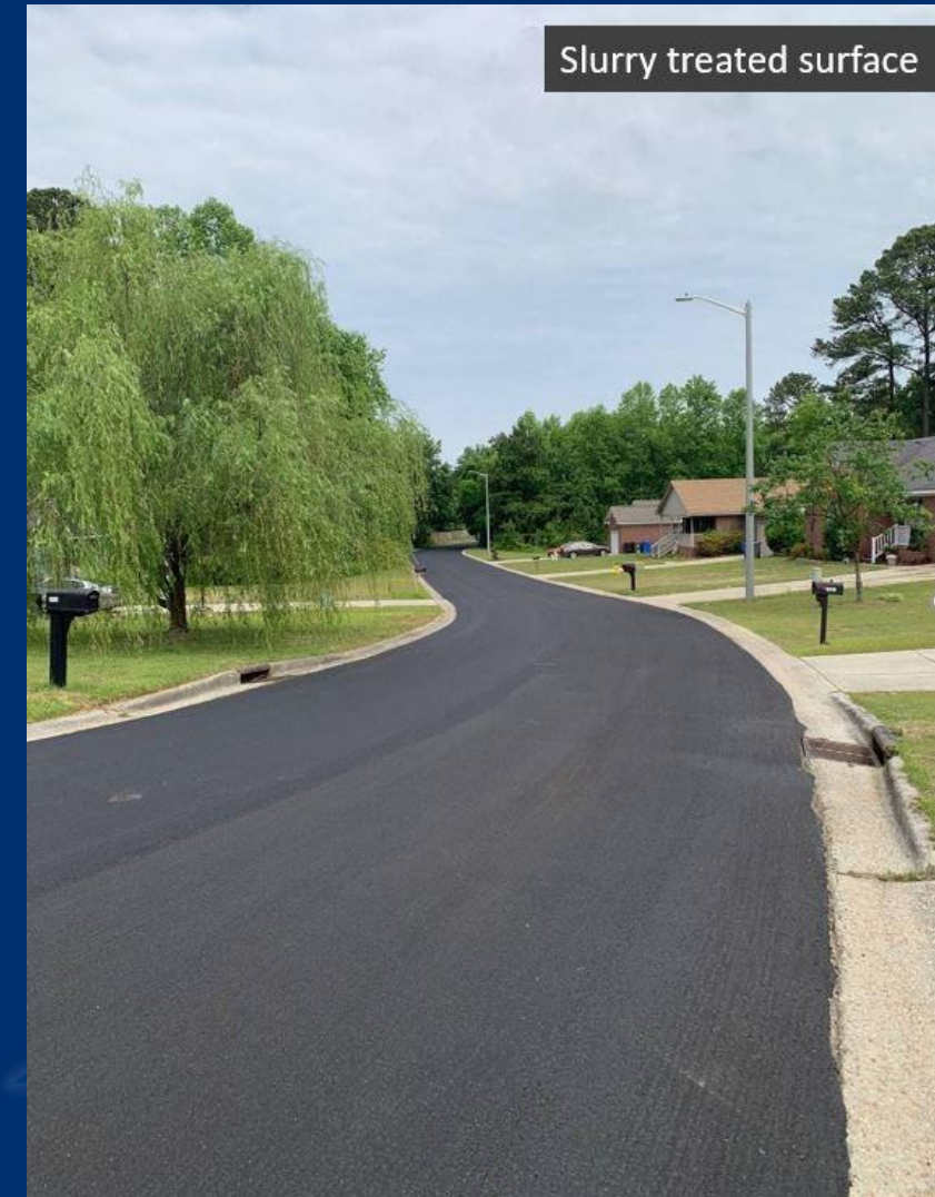
After Surface Treatment
