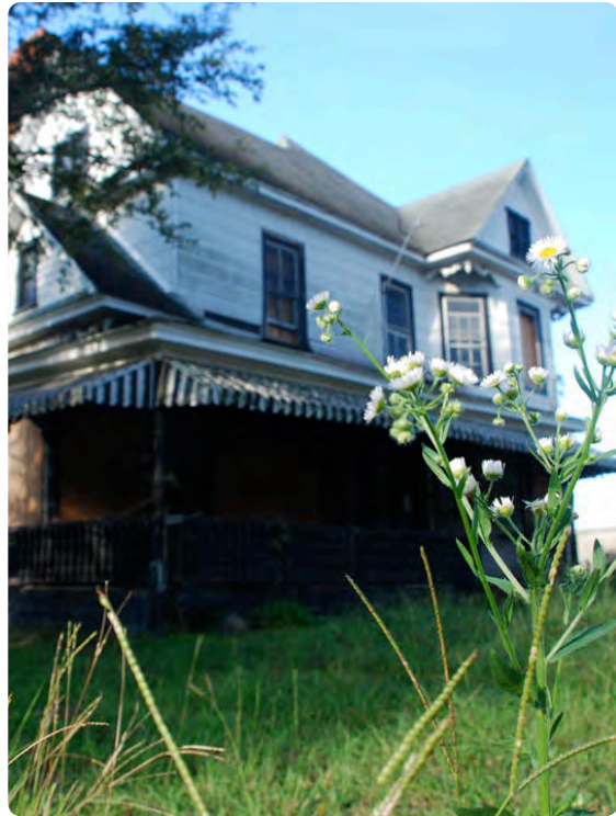
Figure 5.07 – Disused and vacant homes like this one speak to a wealthier time, but gradual reinvestment can help turn neighborhoods in to lively, family-friendly places. (Image source: Studio Cascade, Inc.)
