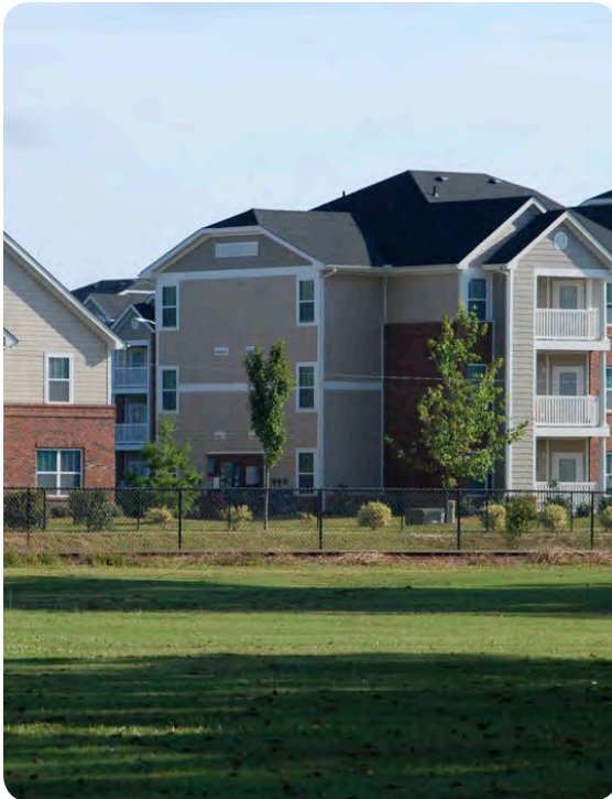
Figure 4.02 – Development at the HOPE VI project north of the Walker-Spivey School has set the bar for quality and intensity. The popularity of HOPE VI demonstrates that mixed-income, mixed-needs housing can revitalize neighborhoods. (Image source: Studio Cascade, Inc.)
