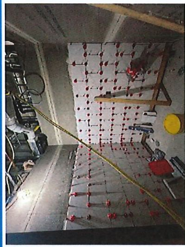
Ceramic tile installation started @ Airline office
