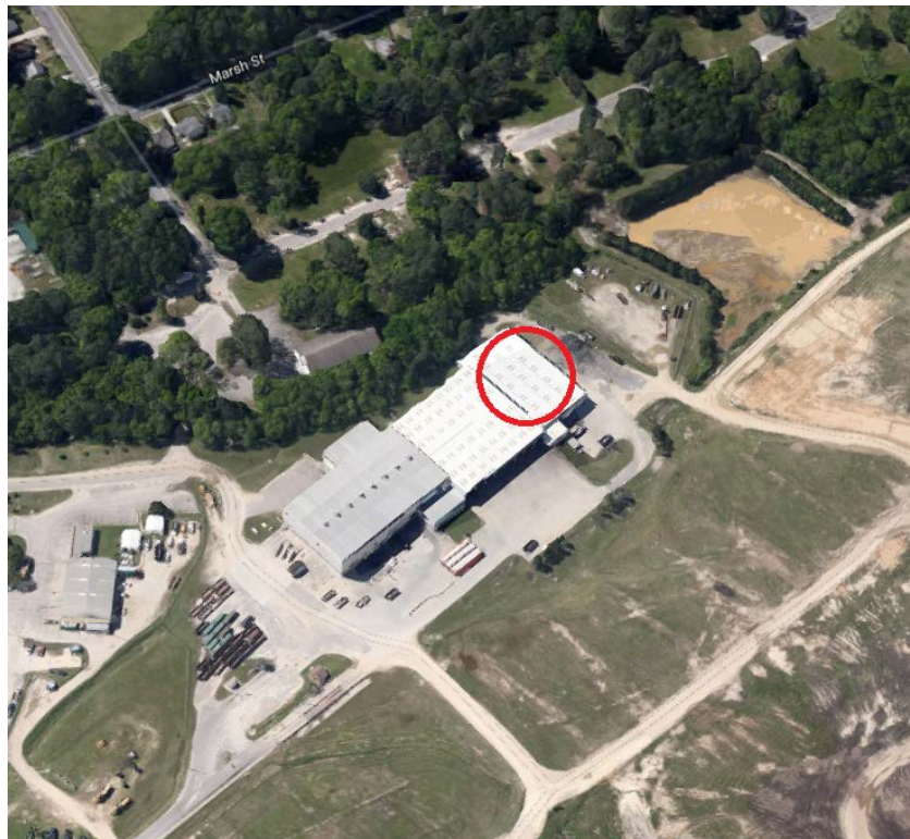
Exhibit 1.1 - Location of Field Sort Site within the BCH Building
