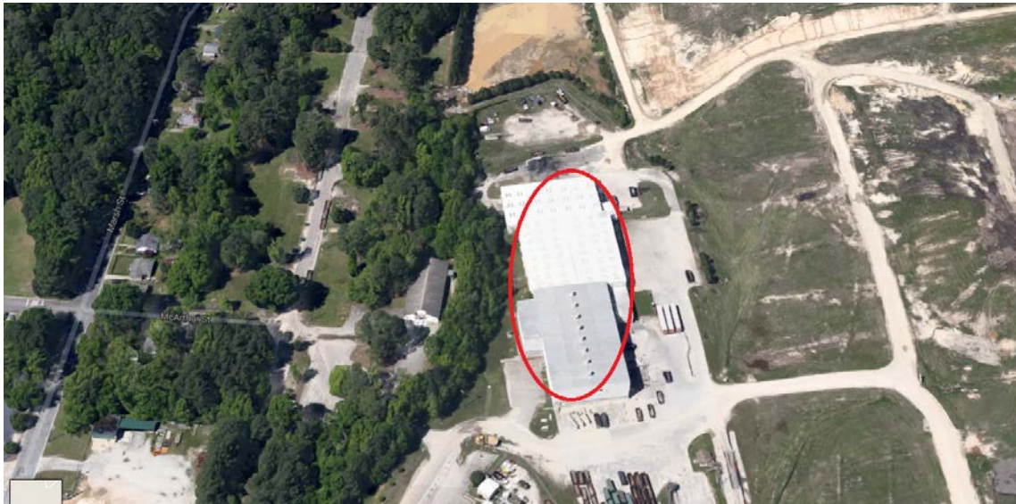
Exhibit 13.1 - Photograph of the Current BCH Buildings at the County Landfill Site
